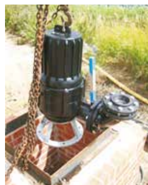
RH80 pump with single-channel impeller installed at Bio-Digester Plant for one of Lincolnshire largest vegetable growers
