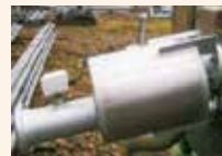
Warmth Exchanger mounted on the pump suction inlet and fitted with a no-flow switch
